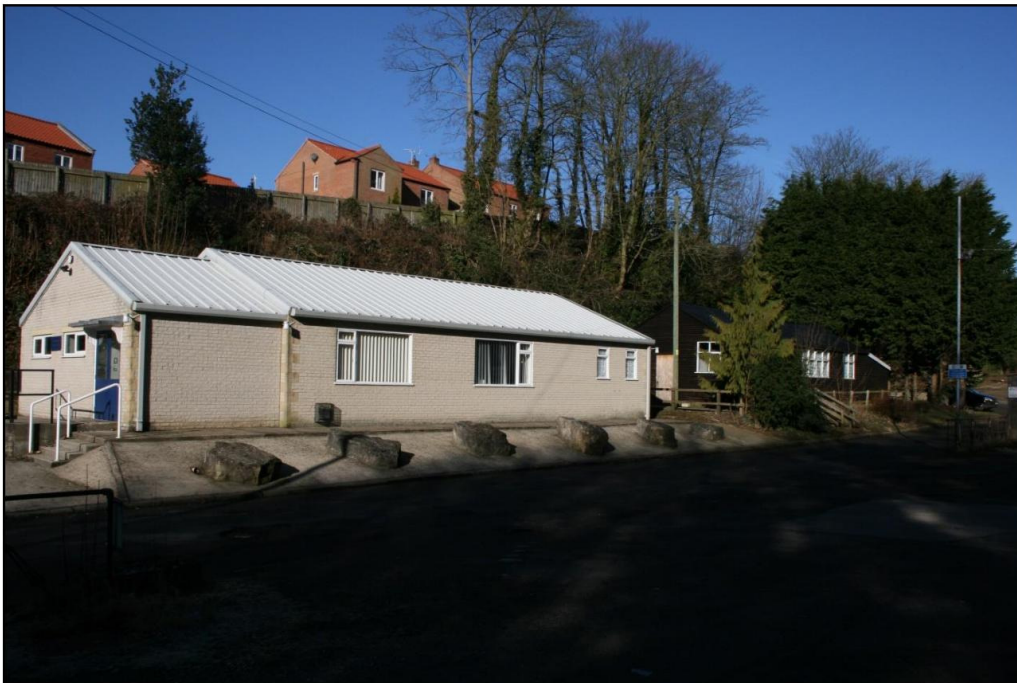
5 Band Hall viewed from development site
