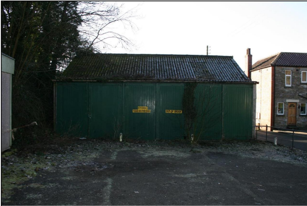
4 Southern section of development site
