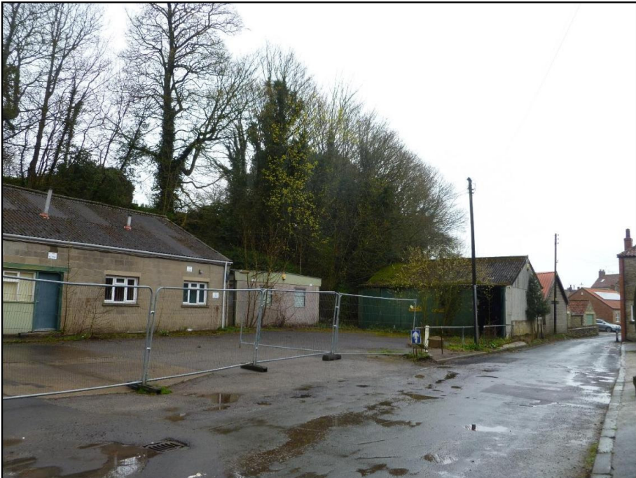
3 Southern section of development site viewed from Manor Vale Lane
